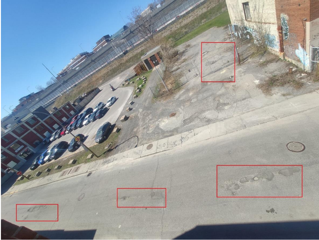
Picture 1 Marks of drilled spots. Photo taken: April 13, 2021
