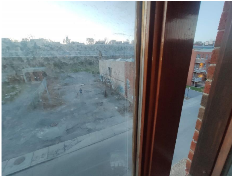
Picture 8 Window dust accumulation after work. Photo taken April 13, 2021, 7.48 PM
