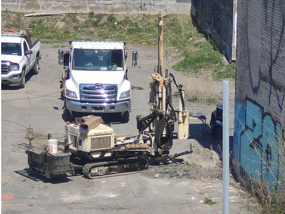
Picture 2 DRILL AND TRUCKS. Photo taken: May 7 2020 10.51 AM
